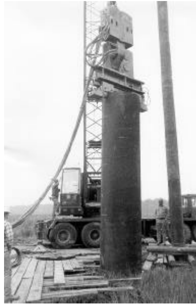
Figure 9 Vibratory Hammer Installing Caissons
