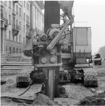
Figure 2 VNIIGS B-402 Vibratory Driver in St. Petersburg, Russia
