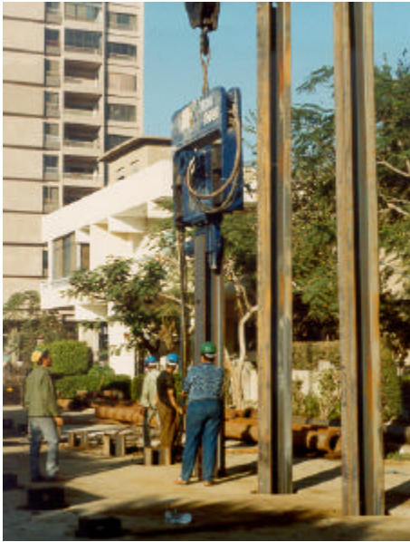
Figure 8 Vibratory Hammer Installing H-Beams
