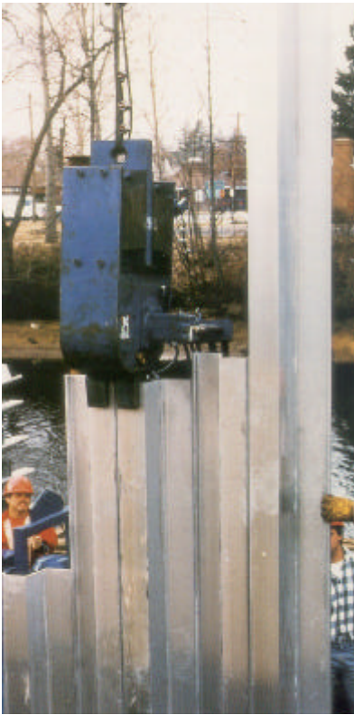
Figure 7 Vibratory Hammer Installing Sheet Piling
