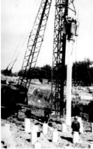
Figure 10 Impact-Vibration Hammer Installing Concrete Pile
